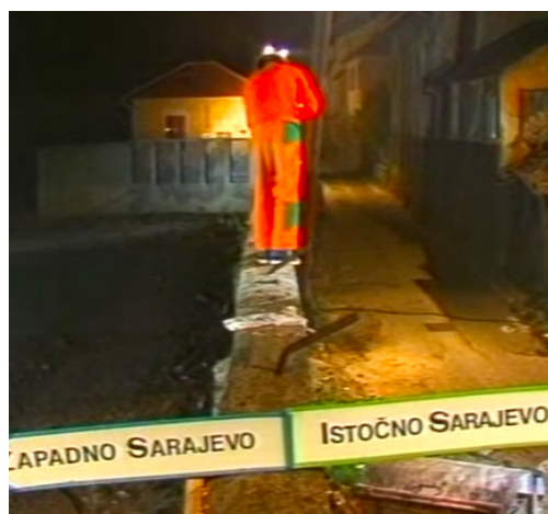
Figure 6.49 Cleaning the wall
